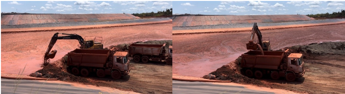
Figure 5. Execution of mechanized cleaning.
