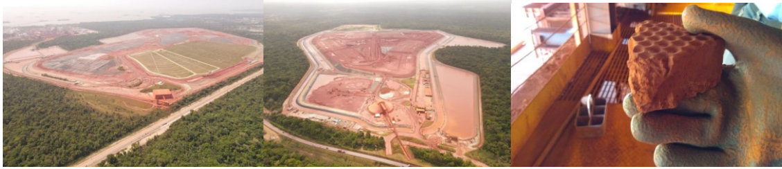
Figure 3. Aerial view of DRS1, DRS2, and the residue cake produced by the filter press, respectively.
