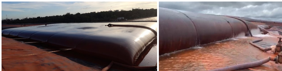
Figure 7. Geobags used at Alunorte in the dewatering process.
